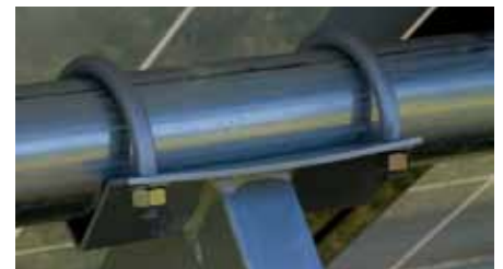
Center right: pipe clamp secures pipe to A-frame
